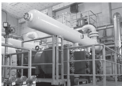
Figure 15 Suction pulsation damper
