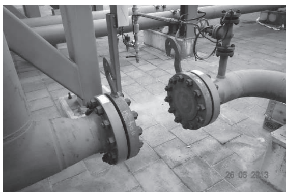
Figure 11. Recycle valve removed for the testing.
