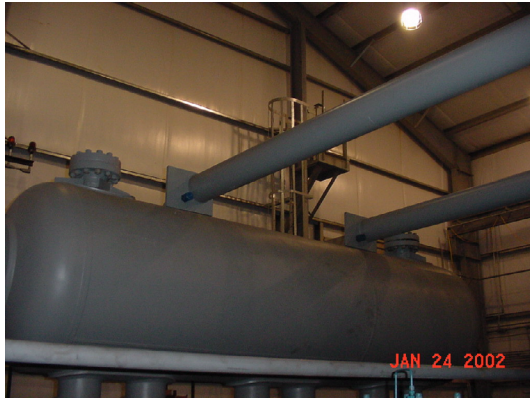
Figure 13. Cross-Brace to Neutralize Opposed Cylinder Excitation of SB Cantilever Mode
