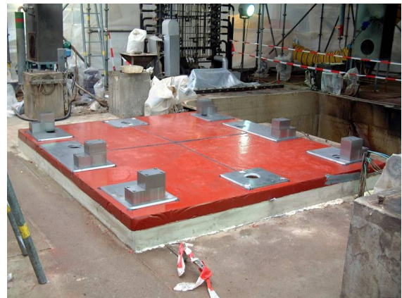
(Picture 3.3.1: Reconditioned Foundation)
