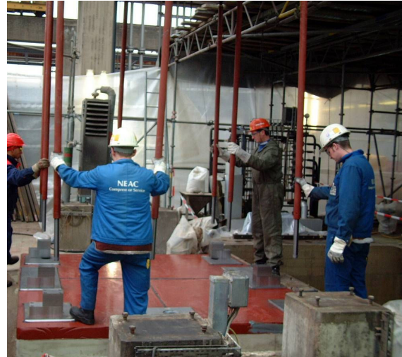
(Picture 3.4.2: Anchor Bolts entering Sleeves)
