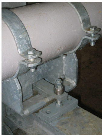
Figure 9: Example of a weight only with a spring hold down support
