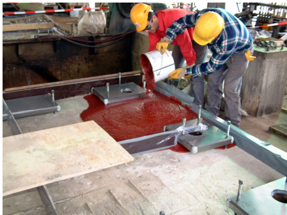
(Picture 3.2.3: Epoxy Grout being poured)
