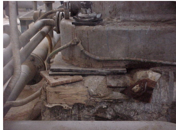
(Picture 1.2: Example of poor Foundation Repair)
