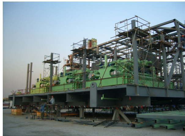
Typical pancake design under Construction
