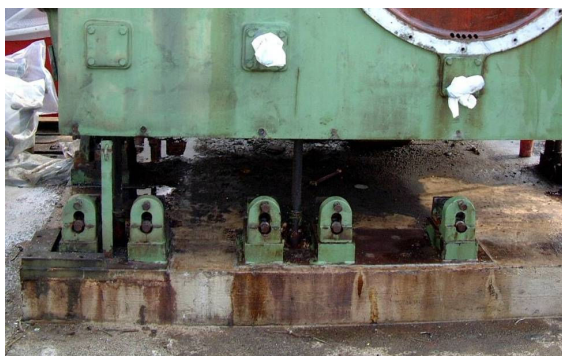
(Picture 2.2.1: Oil Penetration into Foundation)
