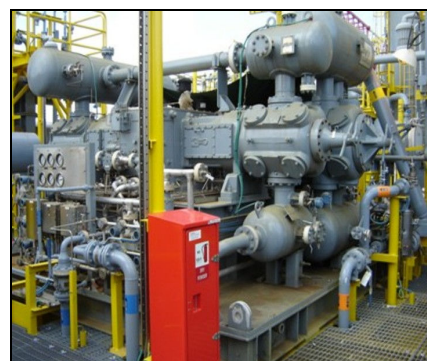
Figure 4: Example of Reciprocating Compressor on FPSO. Dynamic analysis of compressor forces on FPSO structure requires coordination between Machinery Consultant, Packager, and Engineering Consultant
