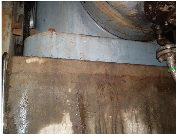
(Picture 1.1: Oil Penetration into Foundation)
