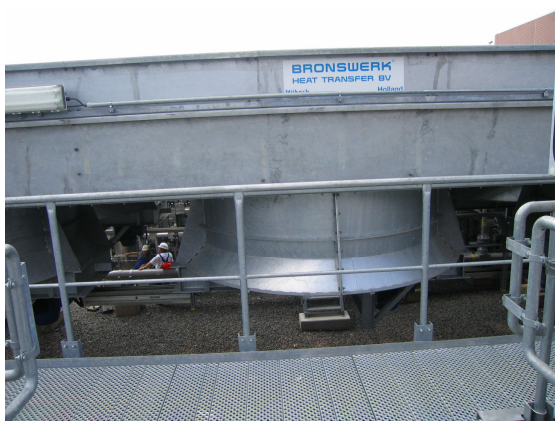
Figure 18: Air-fin cooler
