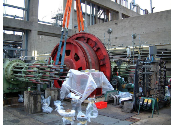
(Picture 3.1: Hyper Unit Disassembly)
