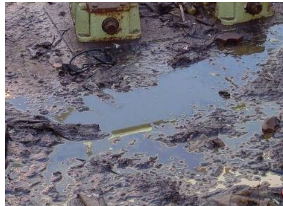
(Picture 2.2.3: Oil Puddle on Top of Foundation)
