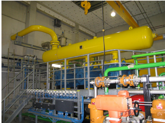
Figure 4: Photo of the suction damper
