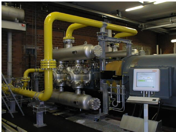
Figure 2: Compressor unit 7 with new installed suction side piping and operation panel.
