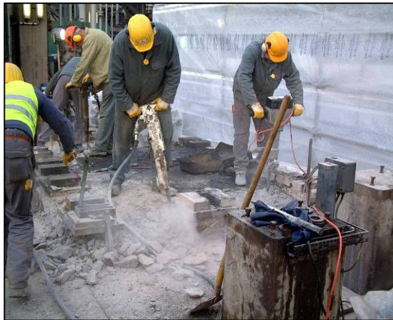
Picture no. 4: Oil contaminated Foundation Top chipped off
