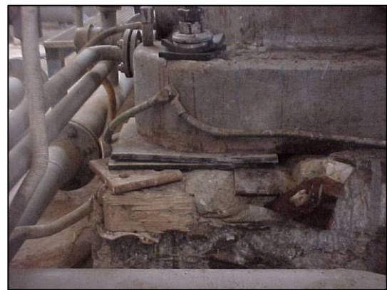
Picture no. 3: Major Damage of Foundation
