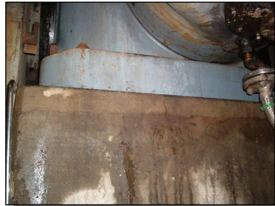
Picture no. 1: Oil penetrated Foundation Block
