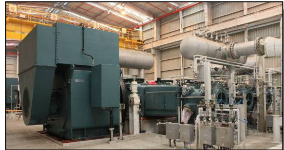
Picture no. 38: 6-Crank NEA Frame Size 500 Compressor
